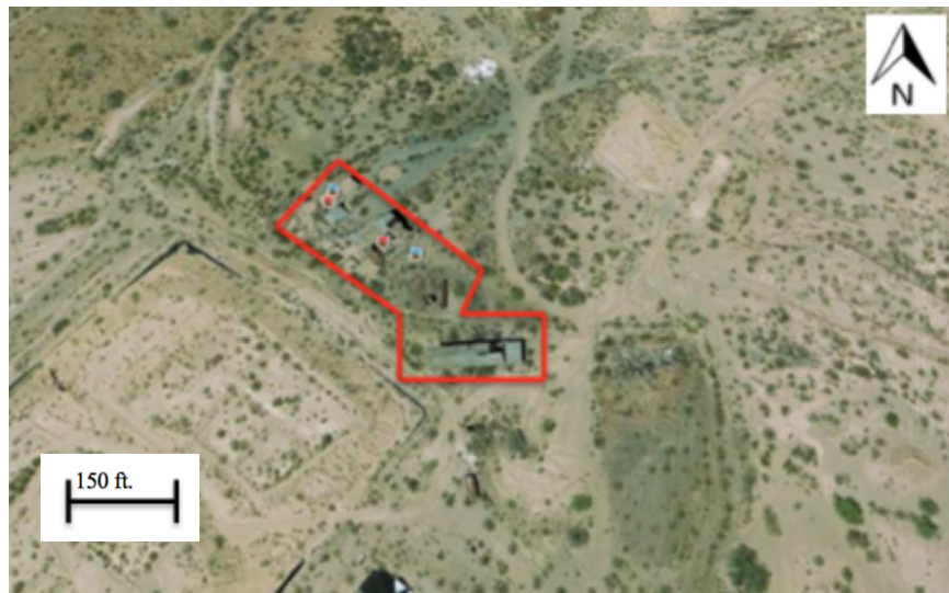
Figure 1.2 Google Earth image of the Vulture mine [3]
